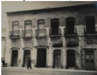
Figura 5 – Rua Riachuelo, trecho entre as ruas Ewbank e Benjamin Constant, 1946
